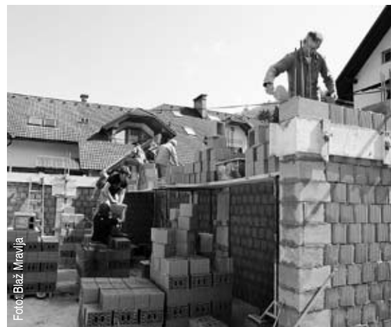
... in gradili nov gasilski dom.
