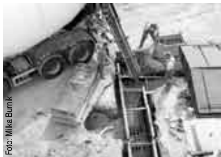
Jet grouting vrtine so globoke 13 metrov
